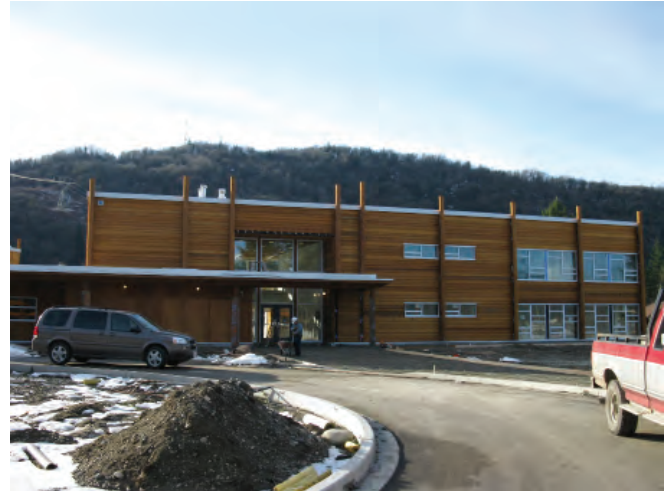
High School Construction 2009
