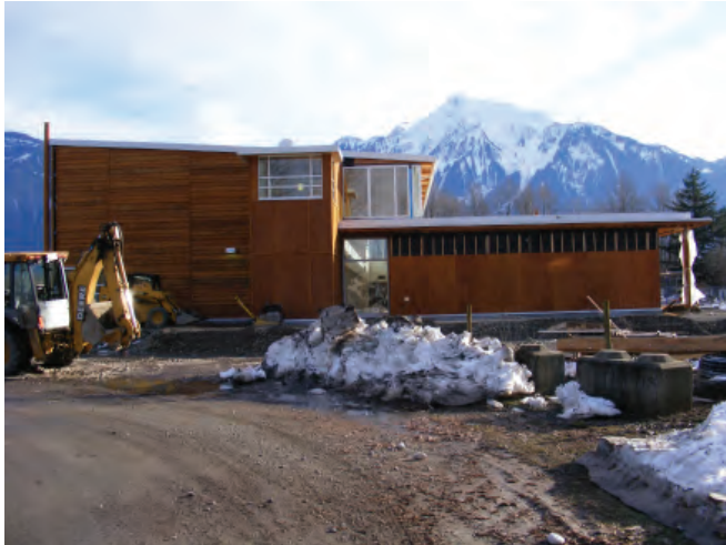
High School Construction 2009
