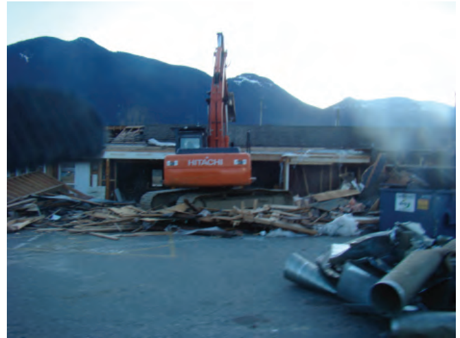
Seabird Cafe Demolition 2010
